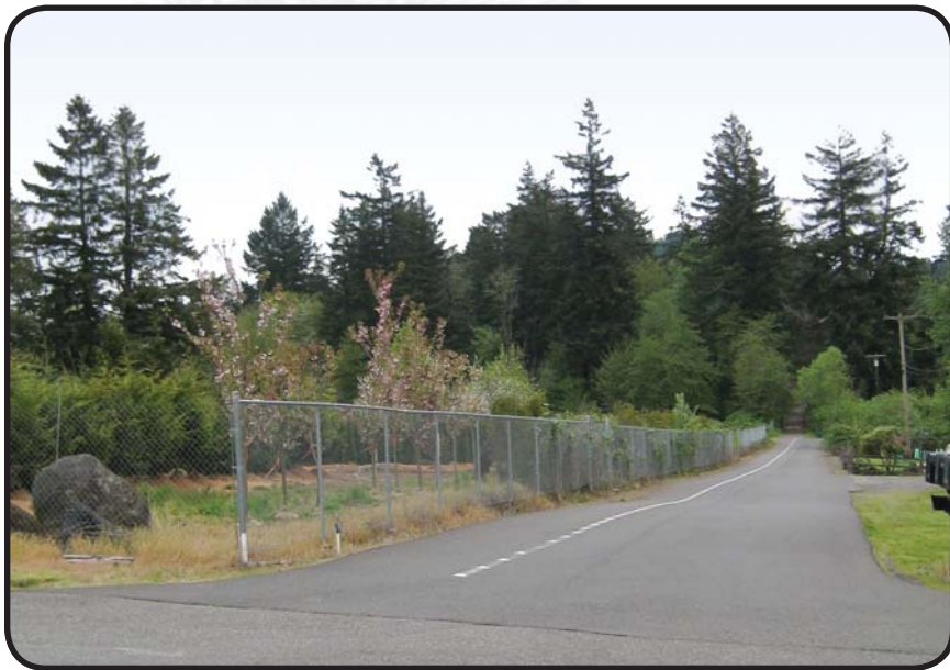
Figure 12. Example of a Widened shoulder with path
