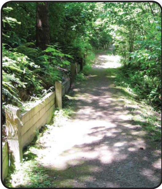
Figure 7. Example of an Uphill Side Retaining Wall
