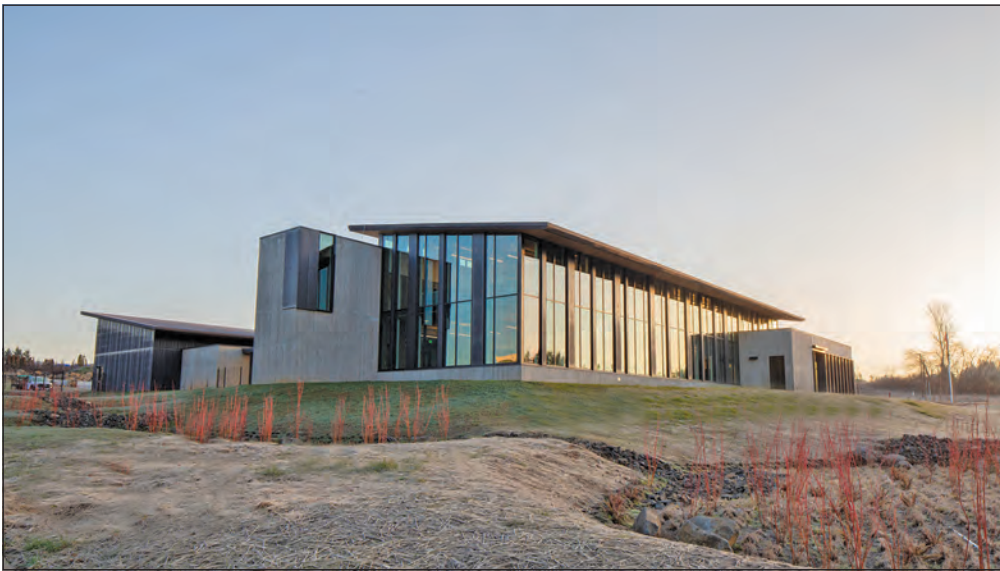
PHOTO COURTESY OF KIRBY NAGELHOUT CONSTRUCTION Kirby Nagelhout Construction's project: Sunrise Water Authority's newest administrative and operations facility.
